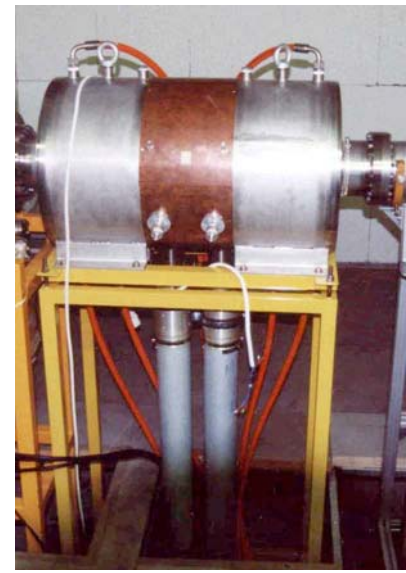
Fig. 43: Power connection with transmission lines
